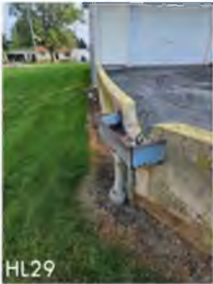
HL29 – Retaining wall at rectory driveway has full depth cracks and leaning.
