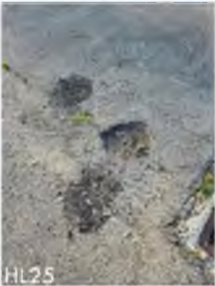
HL25 – Potholed asphalt near drainage structure.
